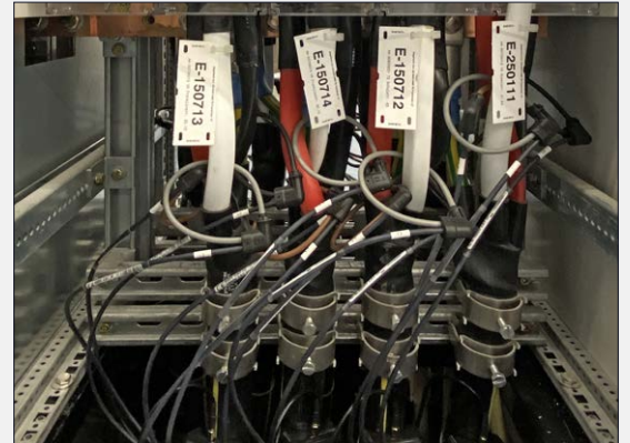
Field installation of Current Link modules
